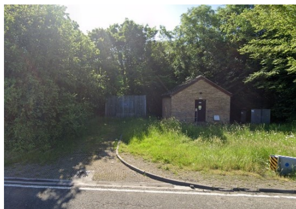
Figure 2-10 Photo of existing TS
